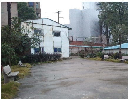
Today there is an empty lot; the parsonage has been demolished.
